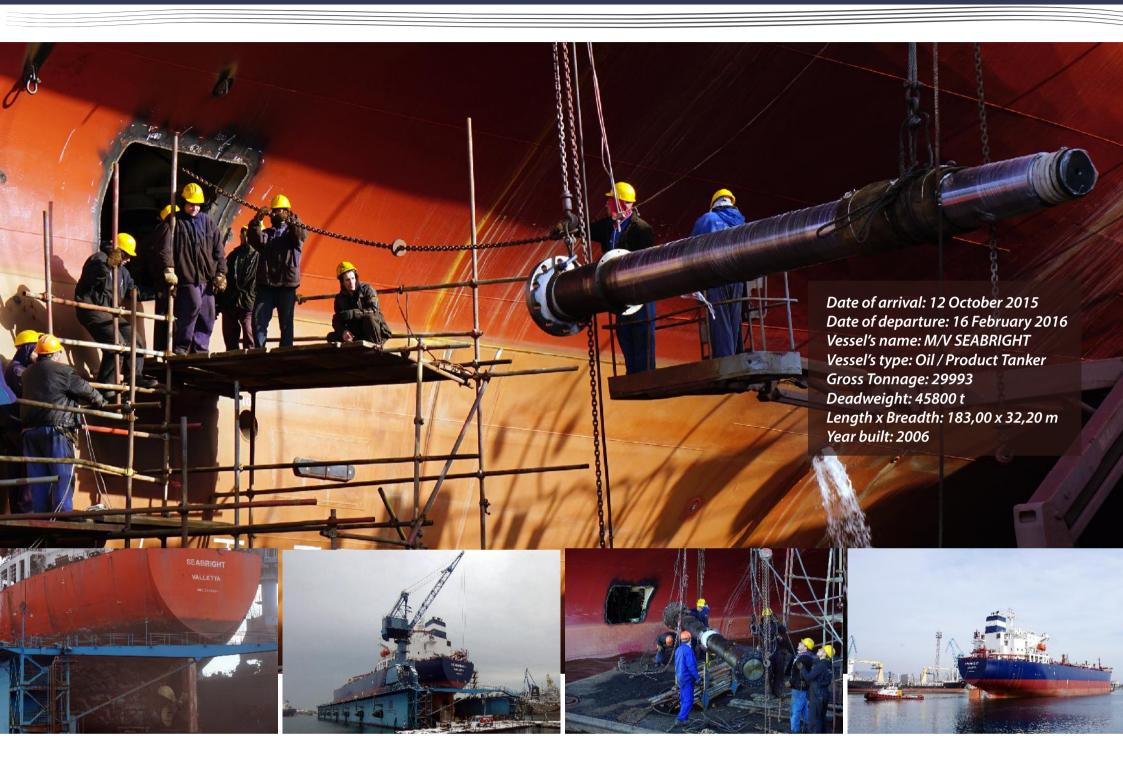
Our longtime, over 22 years client, the major Greek shipping/management company Thenamaris Shipmanagement, chose to award Odessos Shiprepair Yard for repair work to 'Seabright'. She had to carry out standard dry docking, extensive repairs to the tailshaft/ stern tube arrangement (due to bent stern tube, bent tailshaft and destroyed stern tube bearings); also a number of upgrades.
